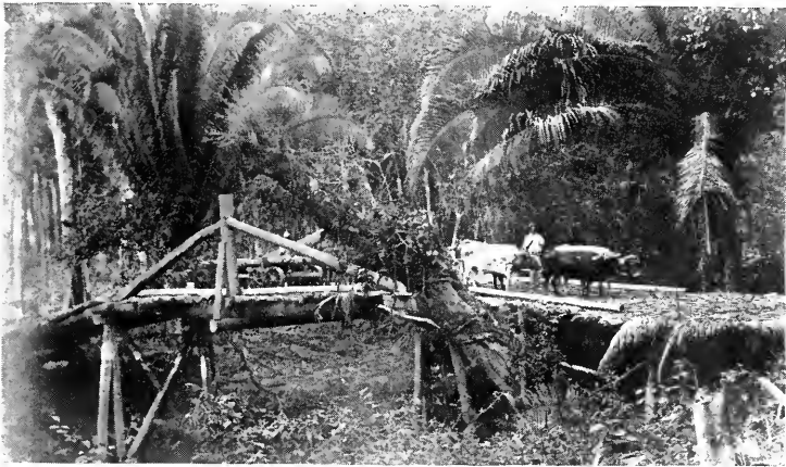
This is the home-made bridge over the Mopan here at San Lorenzo. We are very proud of it. It will bear up to ten or twelve tons without bending too much.
